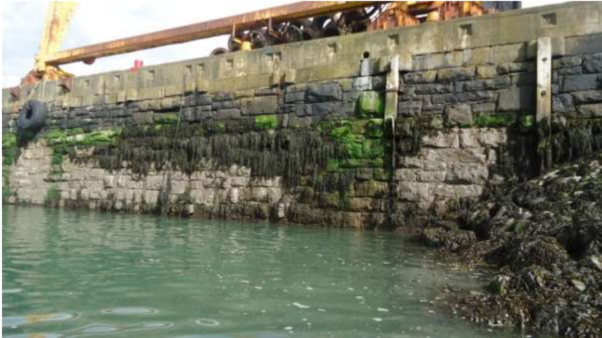
Figure 16.4 View along façade of stone-built quay (ADCO 03) in 2017 before it was buried in the development of Berth 2. The stone work was constructed above the 100-ton blocks that served as the foundation element to the quay.
